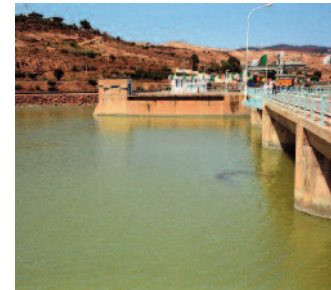
◀ Dam at Fergougue Wilaya de Saida, 400 km West of Algiers
