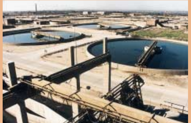
EU-funded Helwan wastewater project, Egypt
