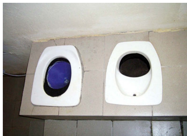
Fig. 5: DESIGN FOR A SEATER URINE DIVERTING DRY VAULT TOILET. ONE SEAT FOR URINE AND FAECES (RIGHT SIDE) AND ONE FOR ANAL WASHING (BURKINA FASO)
