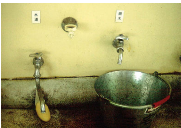
Fig. 7: ▶: MİYAKE ISLAND ELEMENTARY SCHOOL: SUPPLY OF TAP WATER (LEFT) AND RAIN- WATER (RIGHT)
