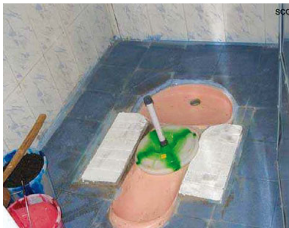
Fig. 3: THREE-IN-ONE SQUATTING PAN DEVELOPED BY SCOPE IN TAMIL NADU
