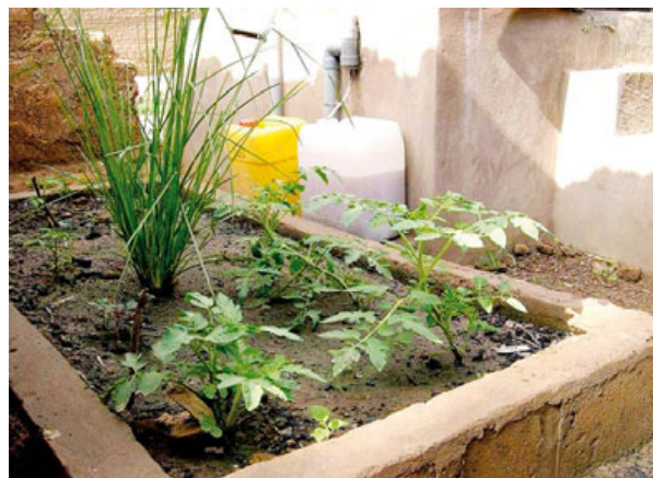
Fig. 6 + Fig. 7: ANAL WASHWATER DRAINED TO A SOAKAWAY (LEFT) AND EVAPO- TRANSPIRATION BED (RIGHT) IN MALI
